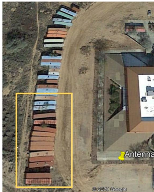
Figure 1: Area where containers will be stacked
