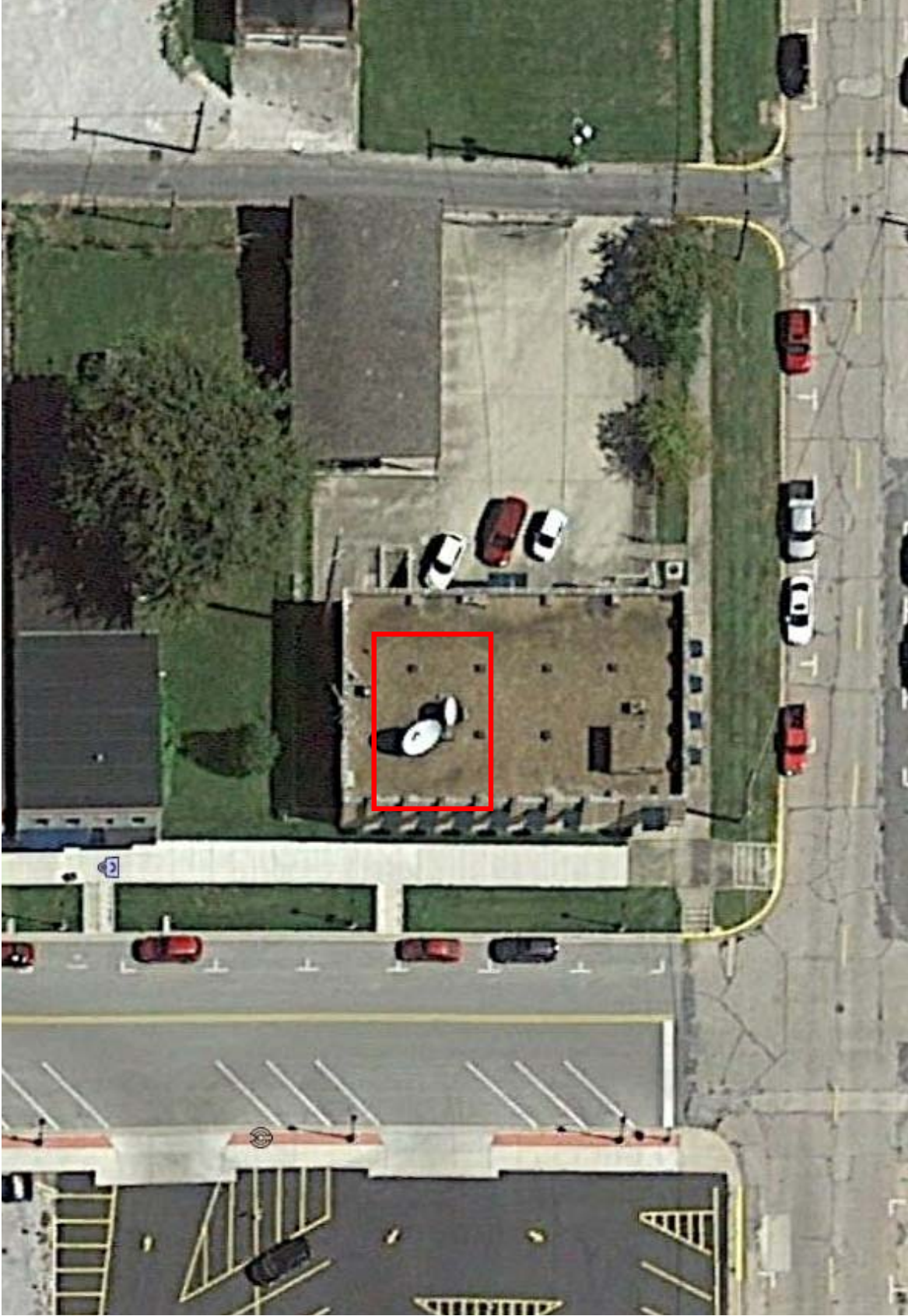
Cromwell Group - WPMB Site, Vandalia, IL 38-57-35.5 N, 89-05-40.4 W (NAD83)
