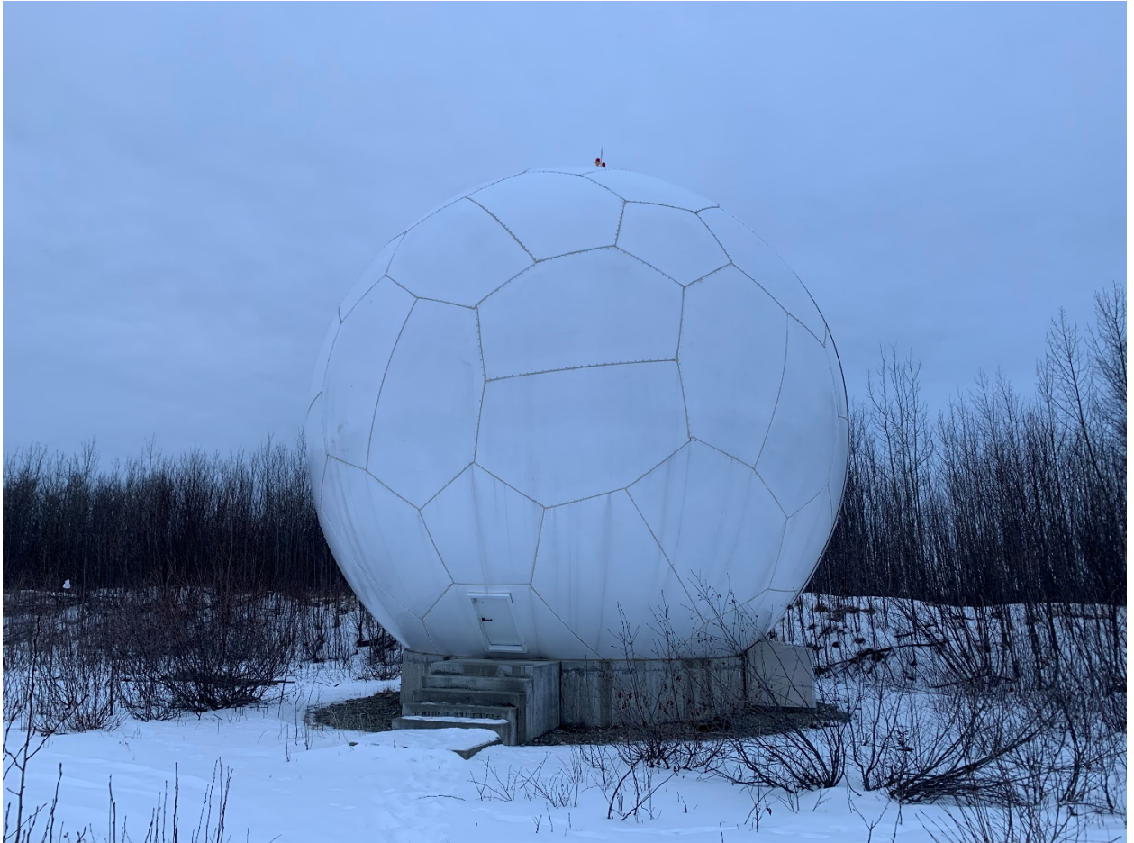
Figure 3. Ground Installation Configuration with Existing Radome
