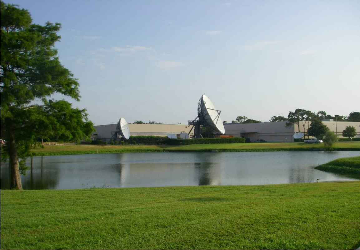
6.3 M Ku-Band Antenna on Left; 13 M C-Band Antenna on Right (both antennas face south east); Building in Back is approx 8.2 M high
