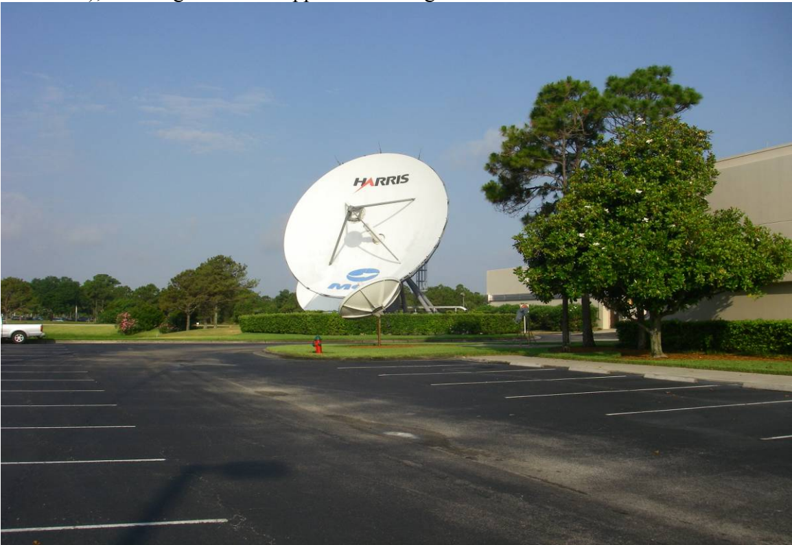
13 M C-Band Antenna pointed SE; Buildings are approx 8.2 M high
