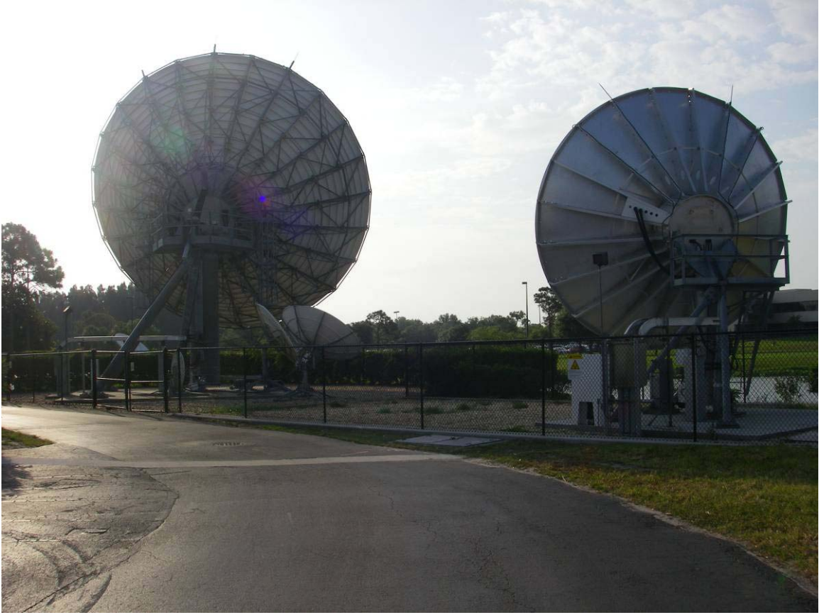
Rear view of 13 M (left) and 6.3 M (right)
