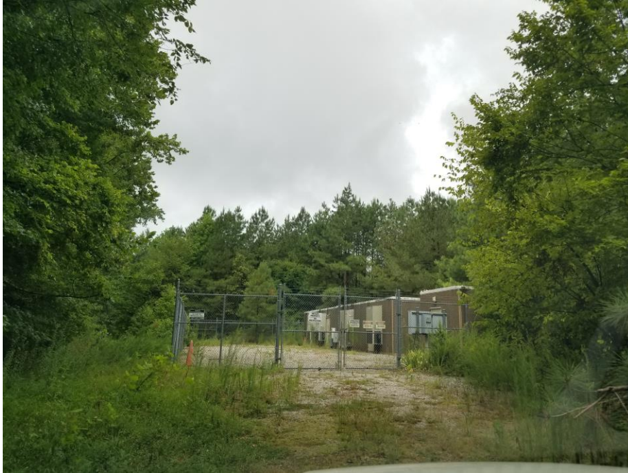
Figure 7: Photos of earth station surroundings obtained during in-person site survey, which preceded earth station construction. Both images taken from the dirt road between the roadway and earth station location, facing westward. These photos demonstrate a mix of deciduous and coniferous trees. This is aligned with the clutter categories of “deciduous trees” and “mixed tree forest” that are being used for PFD contour analysis, and the related clutter assumptions.
