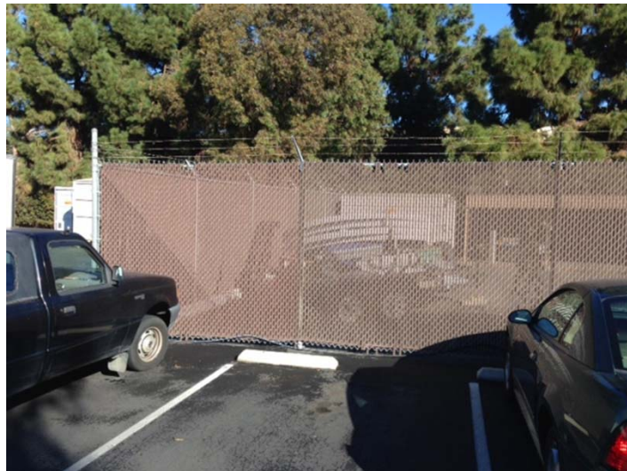
Figure 7. Actual Chain Link Fence Photo.
