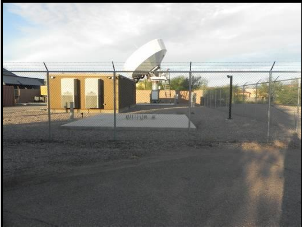
Figure 3.1-1 (cont.) Earth Station Site Photographs
