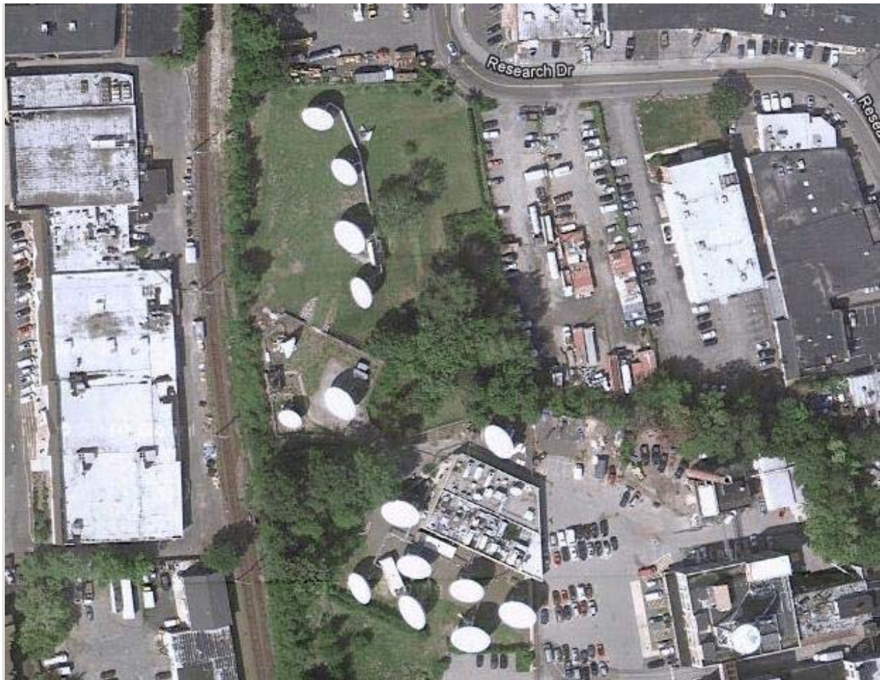
Aerial View of Site
