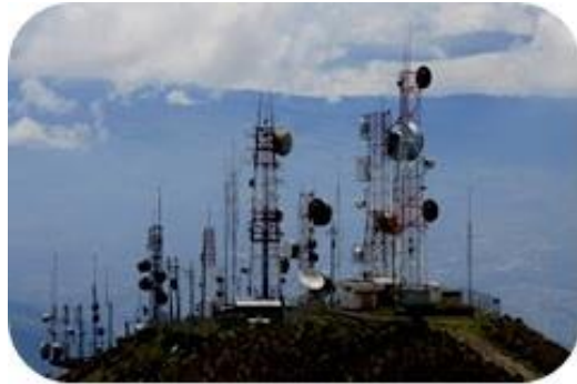
Cell Backhaul and Telecom Trunking
