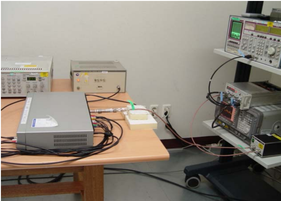
Picture 6. Ant. Transfer Switch
