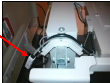
Figure 2. The AC Line Power Sensor Installation Location on the Bed
