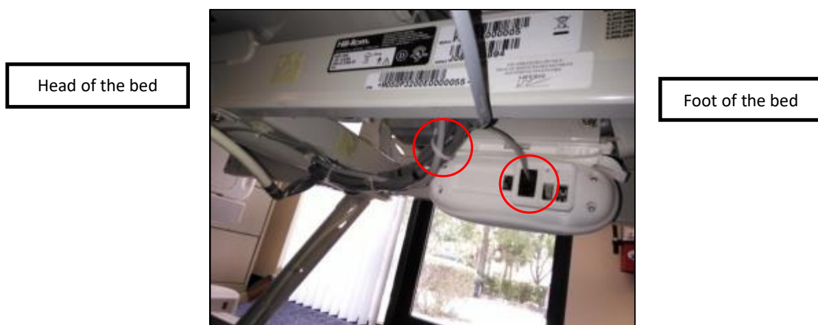
Figure 10. AC Line Power Sensor Cable Routing to Bed Beacon and Cable Tie Holder Placement
