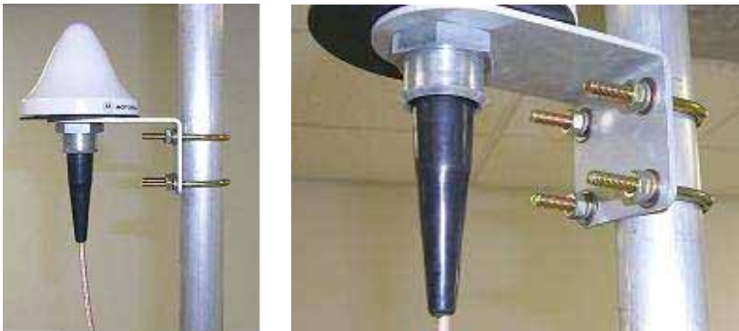
Figure 39 GPS antenna mounting
