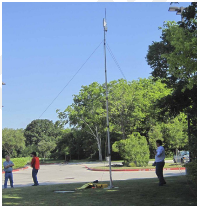
Figure 3–31 Backhaul Antenna Erected
