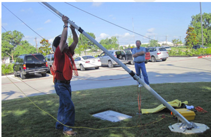
Figure 4–38 Walking the Mast to Vertical 2
