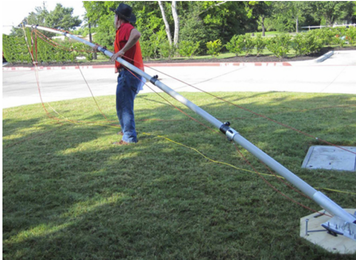
Figure 4–37 Walking the Mast to Vertical 1
