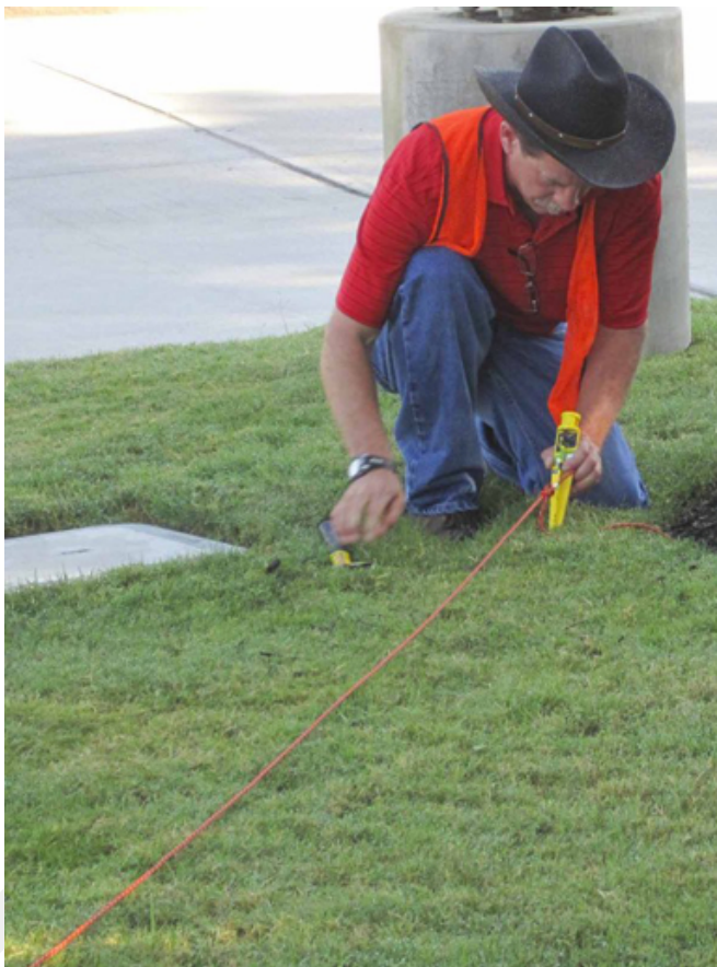
Figure 4–34 Hammering Guy Line Stakes
