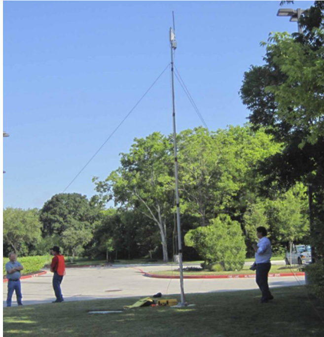
Figure 4–44 Backhaul Antenna Erected
