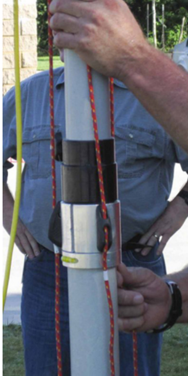
Figure 4–41 Tightening Guy Lines in Cleats
