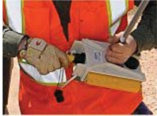
Figure 2–7 Installing the Geophone
