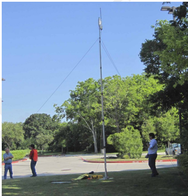
Figure 3–31 Backhaul Antenna Erected
