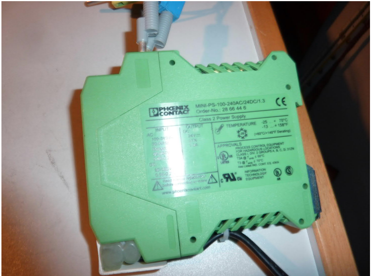
Power adapter MINI-PS-100-240AC/24DC/1.3
