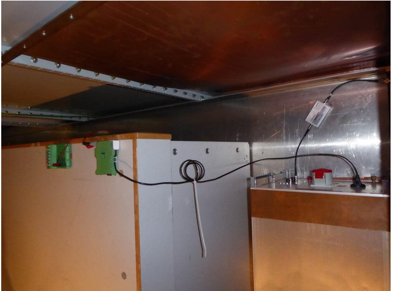
161419_18: Test setup – conducted emissions on power supply lines
