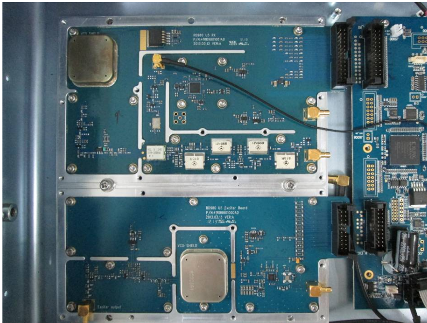
EUT – RX & Exciter Board Cover off View 1
