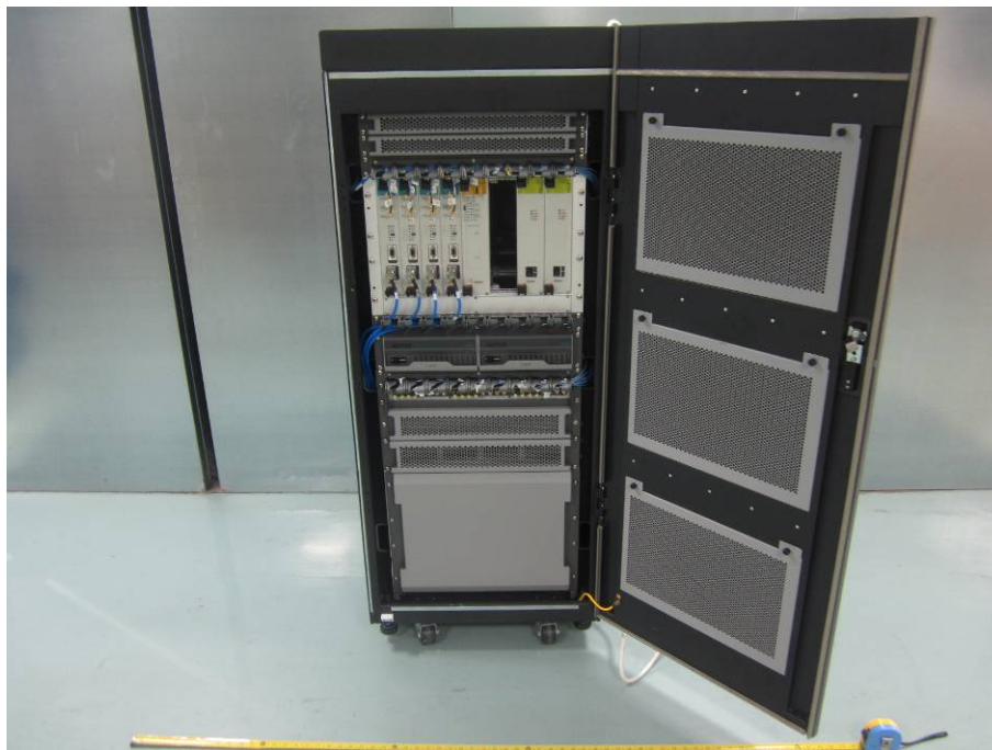
EUT – Front Open View
