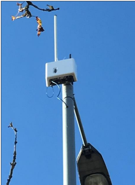
Strap-mount Basestation installation showing power cable connection
