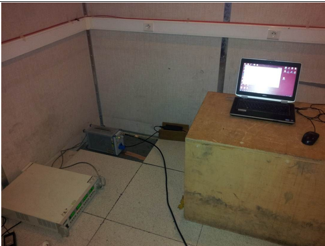
Photograph for AC Power Line Conducted Emissions (Global view)
