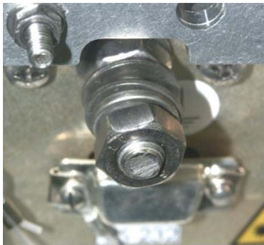
figure 4-7 Grounding bolt with loosened hex nut
