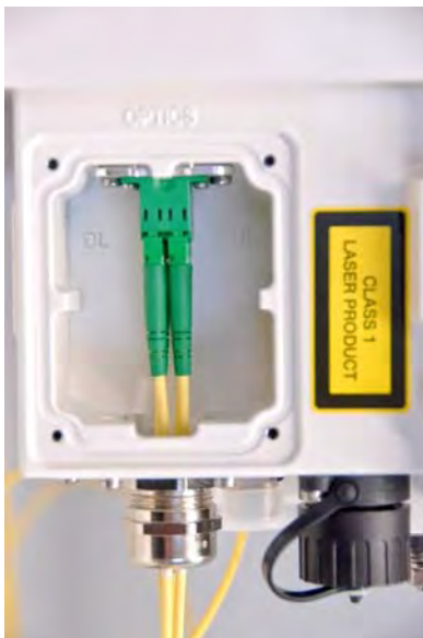
Figure 4-90 Optical cable installed
