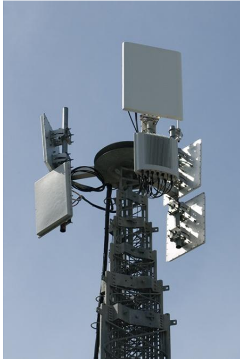
Figure 1: PureWave Quantum 6600 Base Station Mounted on Tower
