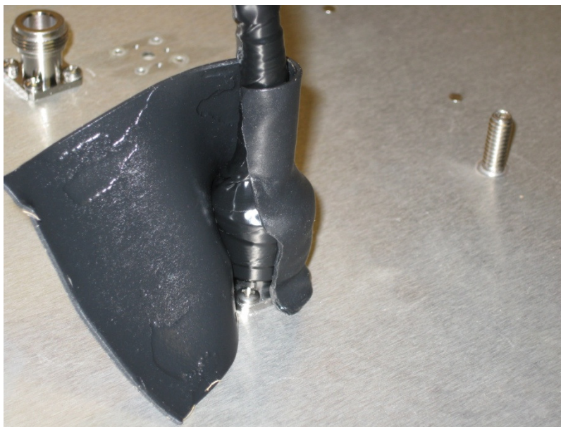
Figure 52 - Butyl Tape Being Applied
