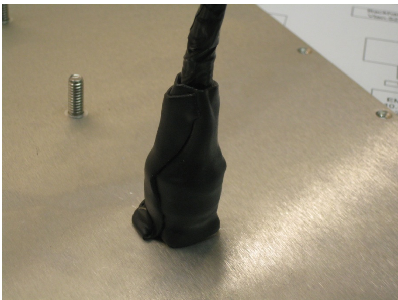
Figure 53 - Butyl Tape Applied
