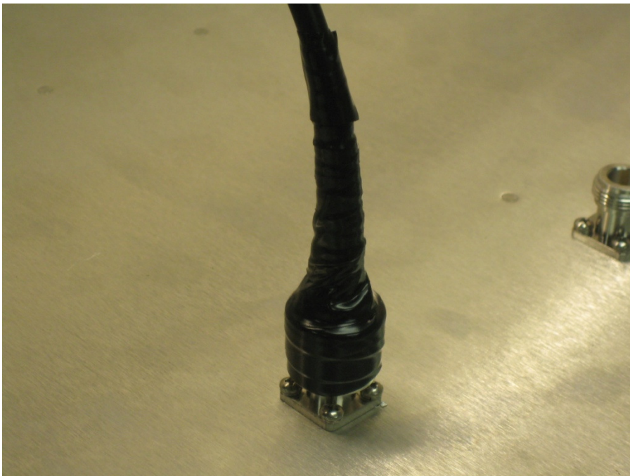
Figure 51 - Plastic (Electrical) Tape Applied
