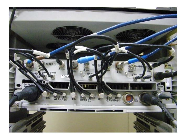
MFRM3 Assembly Front View Fan Assembly Removed
