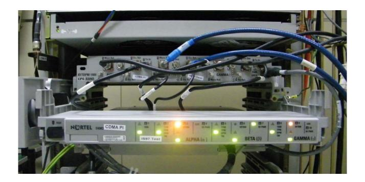
MFRM3 Assembly Front View Fan Assembly Mounted
