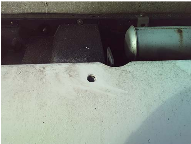
1/2" Hole drilled in Fridge Unit Canopy
