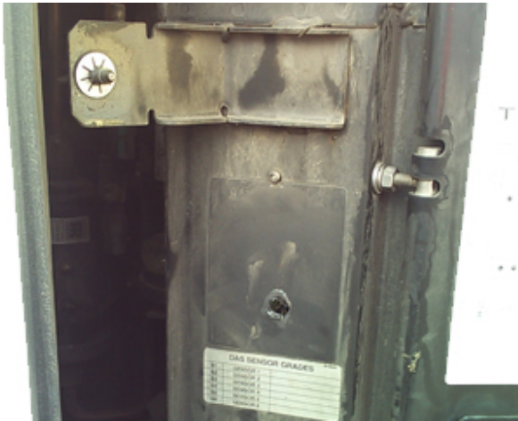
Hole drilled in side of Controller Box for UMD Cables
