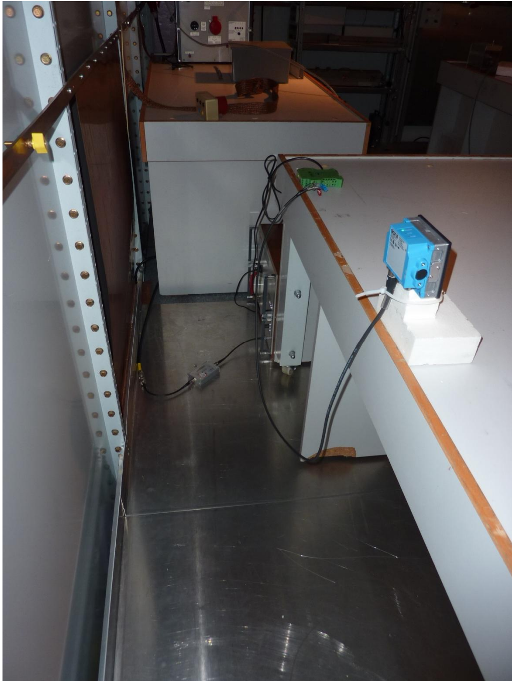
170913_ui.JPG: RMS320-343300, shielded chamber
