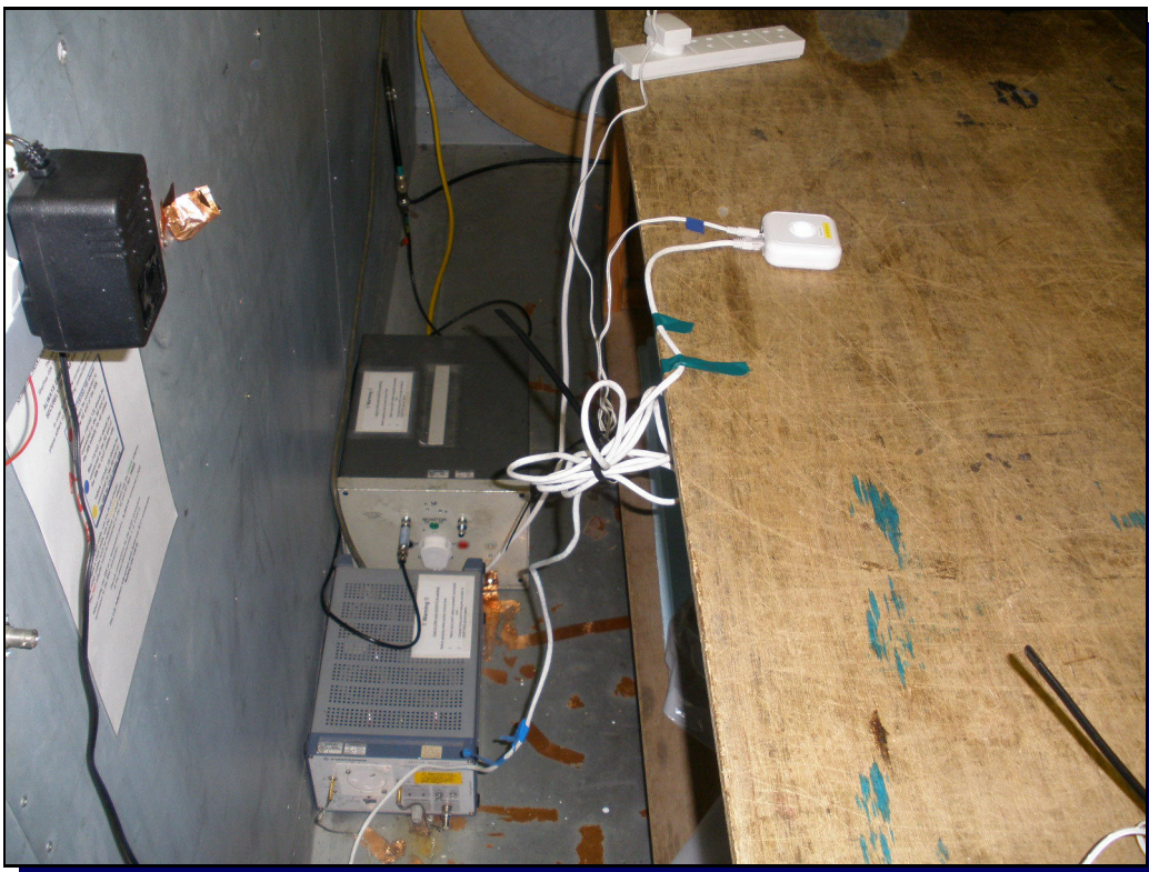
Photograph 2 Conducted Emissions - Back
