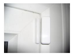
Or, you could try adding a spacer (such as a bit of plastic, or a section of an old credit card) to move the magnet part of the sensor:
