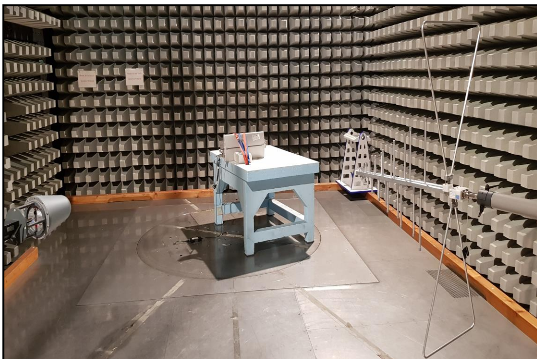
Photo 10: ARU 3500 +WIRA-30-circular-FCC Antenna
