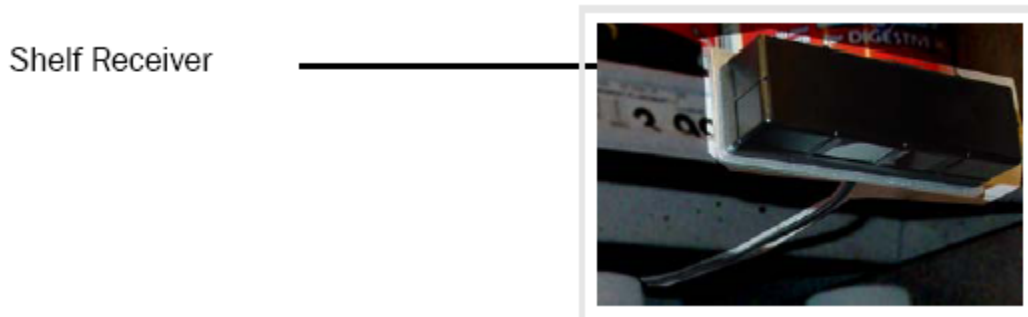
Figure 13. Installed Shelf Receiver
