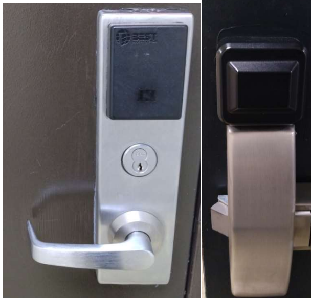
Inside escutcheon (antenna location)
