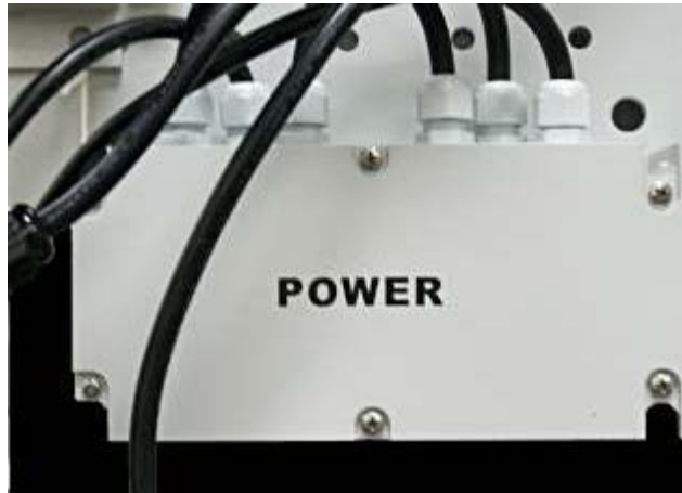
Figure 35 AC Power Junction Box
