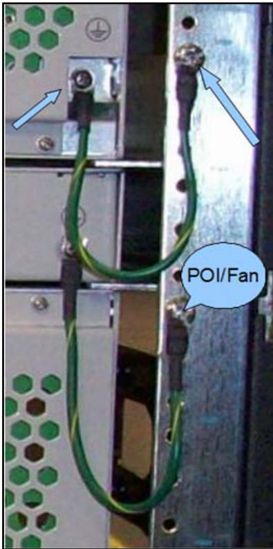
Figure 4-16. Grounded Host Unit (shown with optional POI Unit, also grounded)
