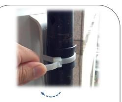
Step 4 Using the clockwise pulling force to ensure it has been completely tighten and locked.
