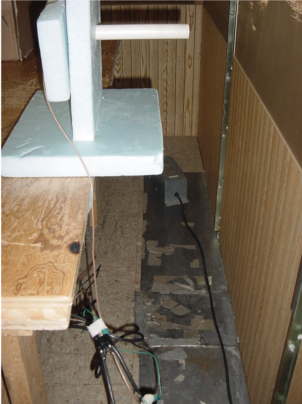
Photo Description: DC Line Conducted – Back
