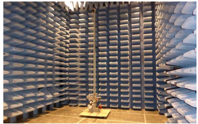
5 m Semi-Anechoic Chamber (SAC) in Everett, Washington
