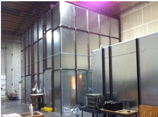
5 m Semi-Anechoic Chamber (SAC) in Everett, Washington
