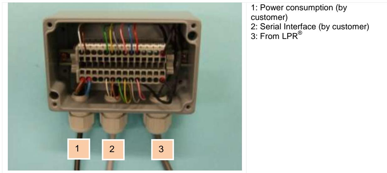
Figure 13 Example for wiring connector box with 8 pins
