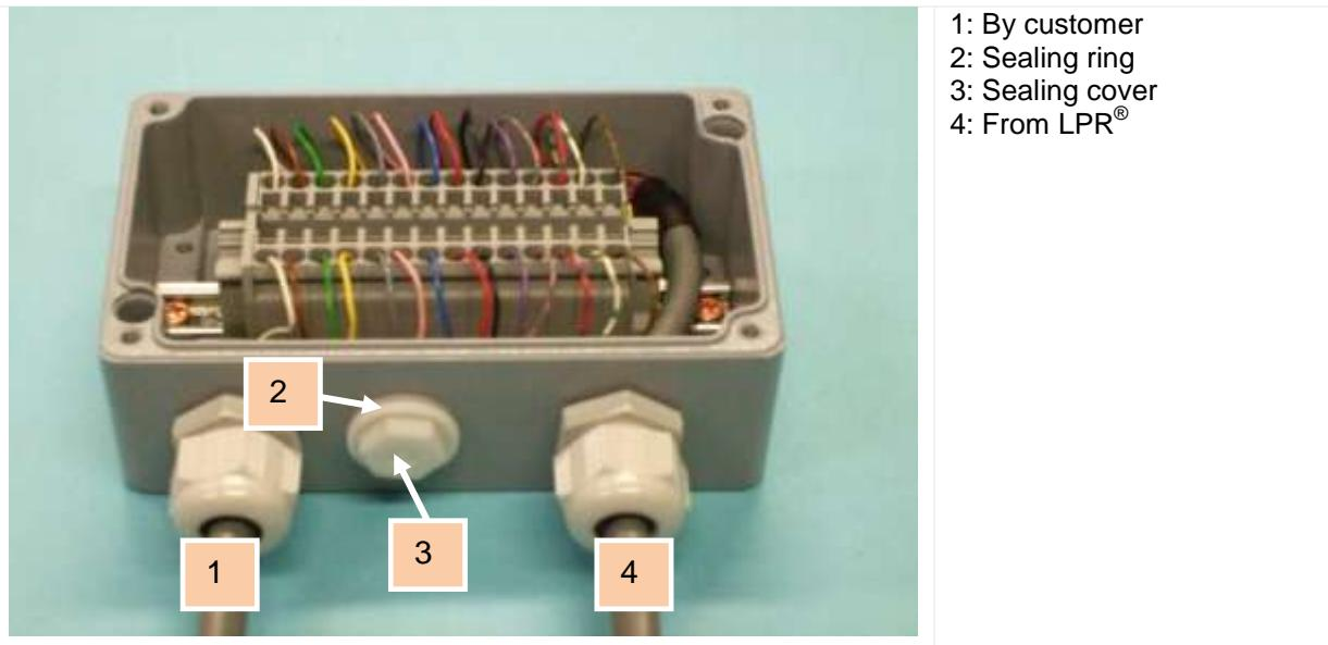
*Figure 14 example for wiring of connector box with 14 pins*
