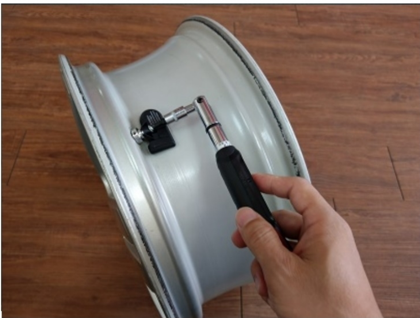
Install sensor. Adjust the sensor to fit the drop well of the wheel. Use wrench to keep stem vertical then tighten. Tighten the screw until 2.2Nm (Recommended Final Torque Setting)
