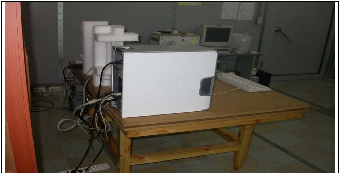
Figure 2 : Rear for NEC Panel
