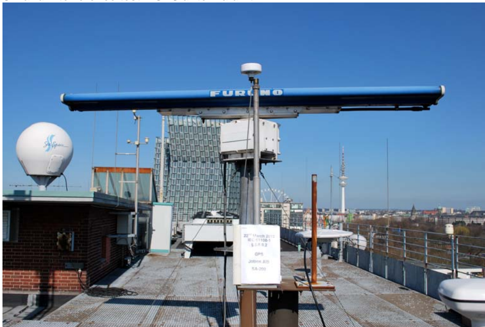
S-Band interference test – GPS antenna unit 1
