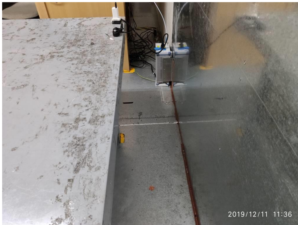
Photograph 10: Set-up for AC Mains (Back View)
