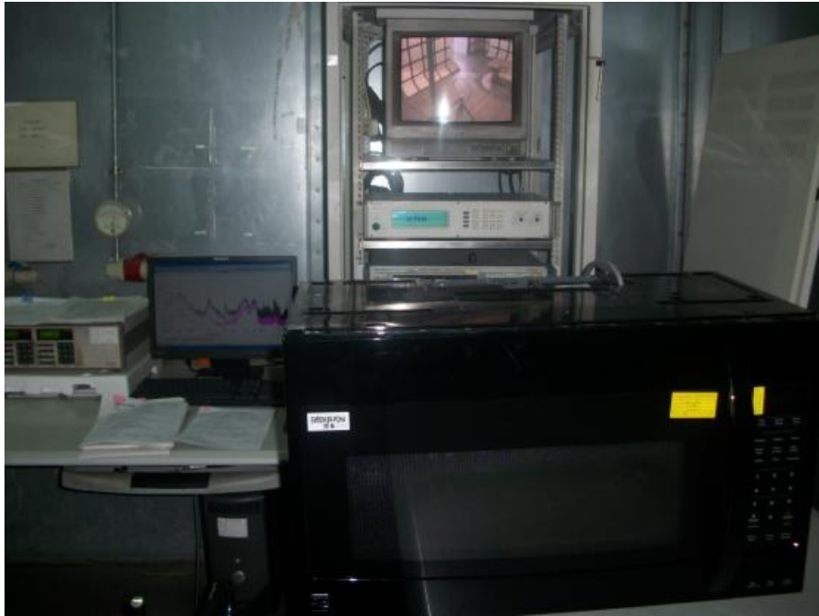
Conducted Emission Test Set-up
