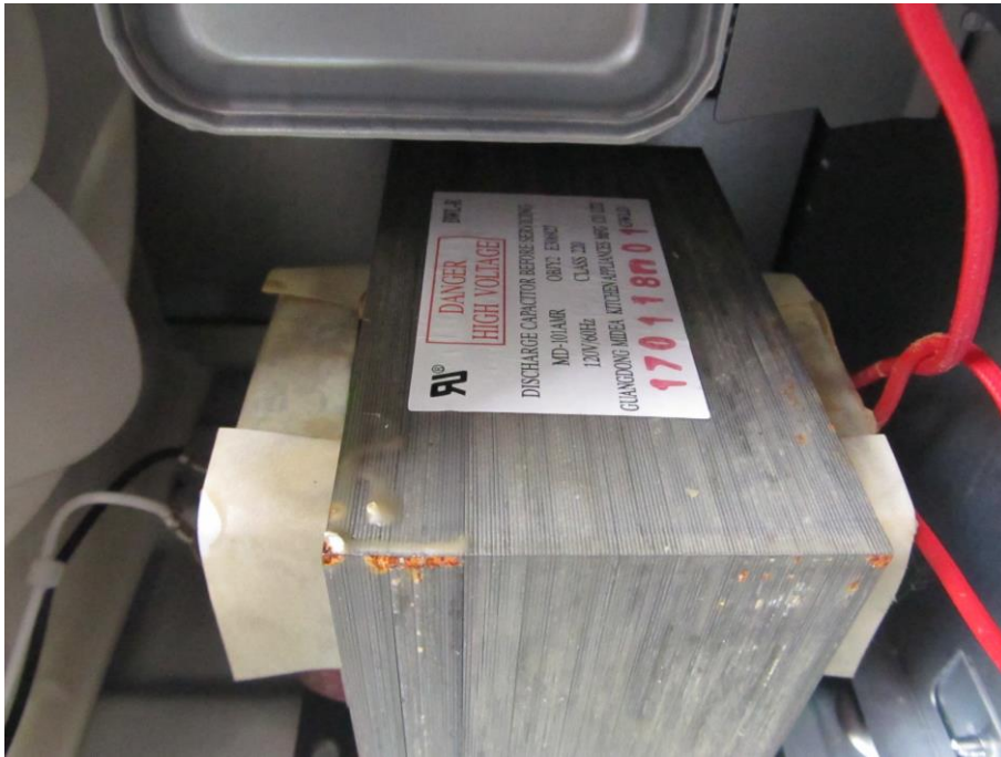
High-voltage Transformer View
