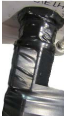
Figure 19: Wrapping the Connector with Electrical Tape
