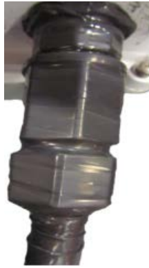
Figure 18: Wrapping the Connector with Rubber Splicing or Self-Amalgamating Tape
