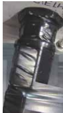
Figure 4.7. Wrapping the Connector with Electrical Tape
