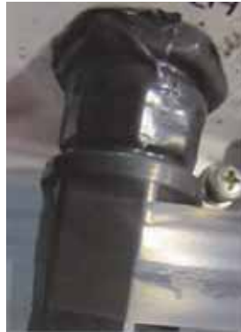
Figure 4.5. Wrapping the Connector with Rubber-splicing or Self-amalgamating Tape
