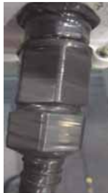
Figure 4.6. Wrapping the Cable with Rubber-splicing or Self-amalgamating Tape
